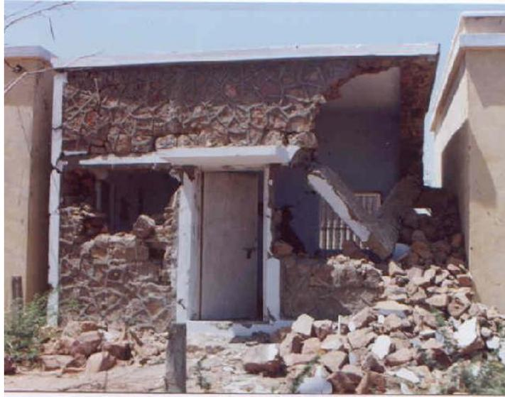
**Plate 4: Local failures**
