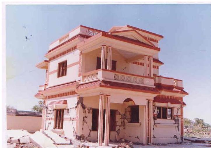
**Plate 10.6: In-plane shear failure**
