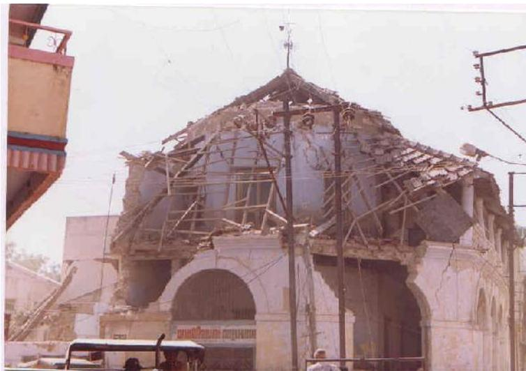
**Plate 1: Out-of-plane flexure failure**
