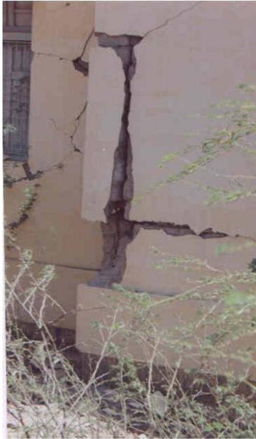
**Plate 2: Separation of wall at junctions**
