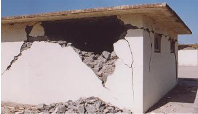
**Plate 6: Separation of roof from walls**
