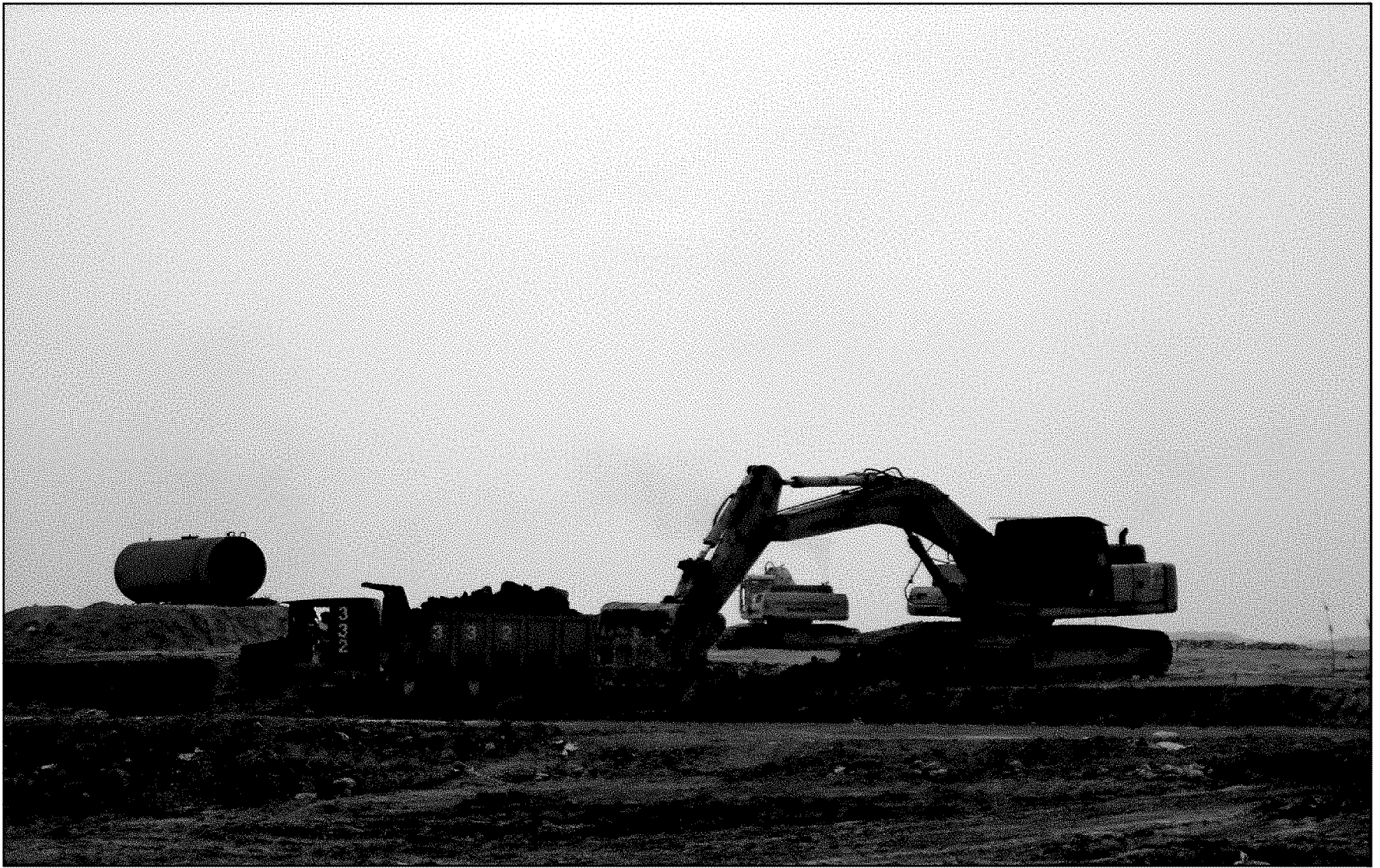
Excavator heaping up top soil
