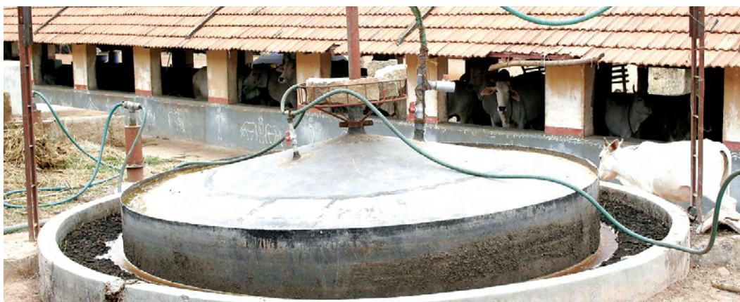
Fig.3.11-Biogas (Gobar gas) plant
