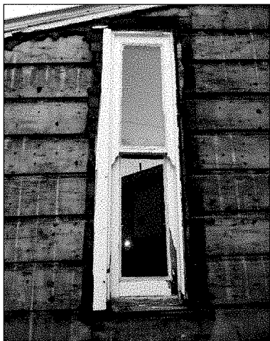
Removing later materials may reveal the original materials, such as this siding, which with care can be successfully repaired.
