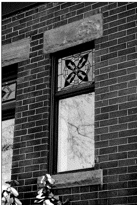
Matching the existing brick pattern or bond and the composition of the mortar help to ensure the integrity of the brick and stonework and consequently architectural character.
