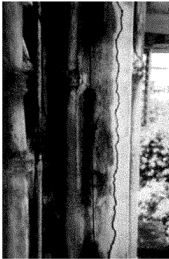
Crack formed due to bursting pressure on account of rusting of reinforcements
