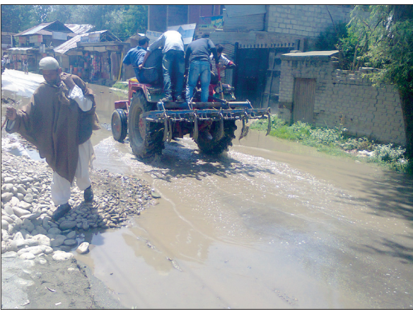
The dilapidated condition of Haigam market road caused by blocking of drains. Majid Kambay (Haigam, Sopore, Baramulla)
