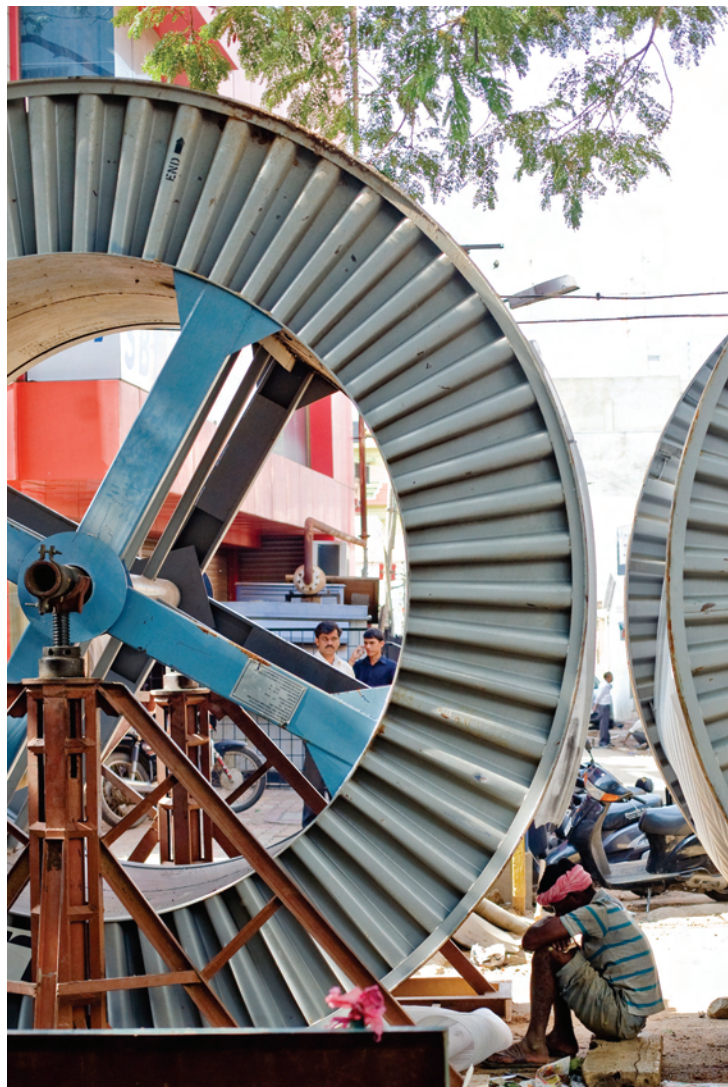
Fig 19.4 Workers laying cables
