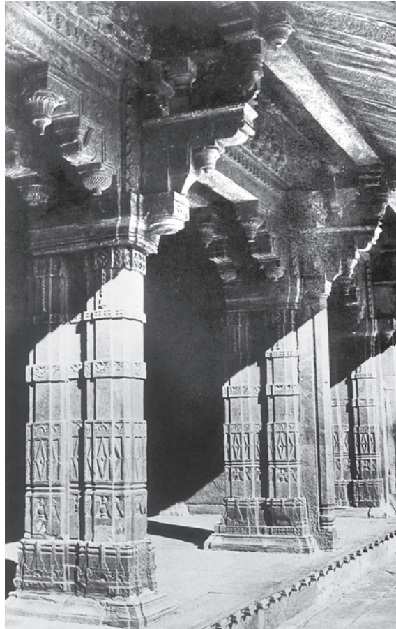
Fig: 22.16 Decorated pillars and struts holding the extension of the roof in Jodh Bai palace in Fatehpur Sikri. They follow the architectural traditions of the Gujarat region.
