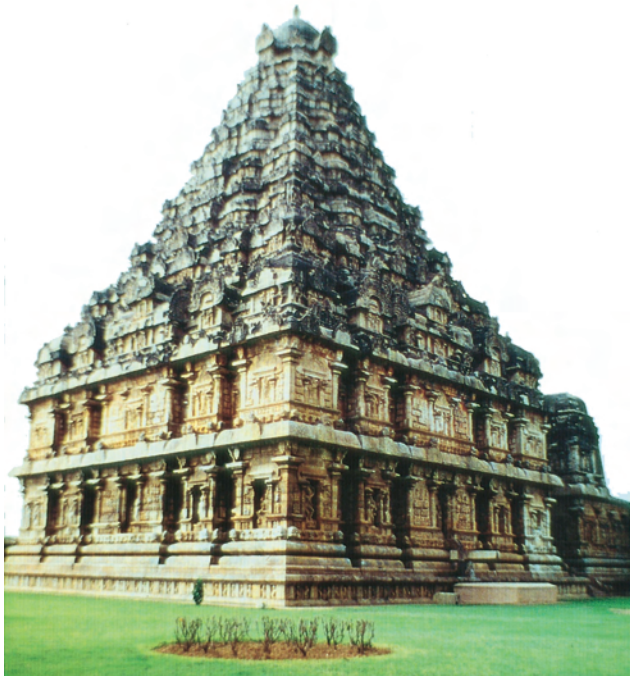
Fig 11.3 The temple at Gangaikonda-Cholapuram. Notice the way in which the roof tapers. Also, look at the elaborate stone sculptures used to decorate the outer walls
