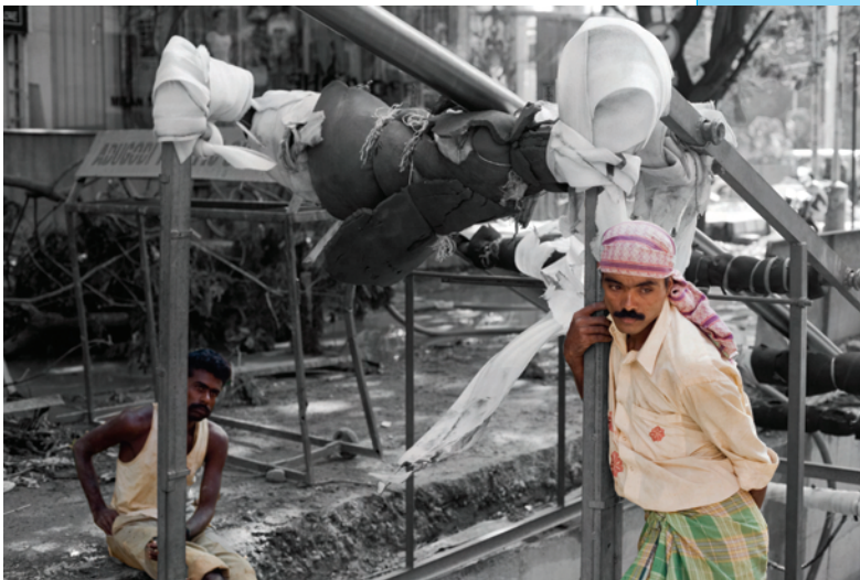
Fig 19.5 Road Laying Work
