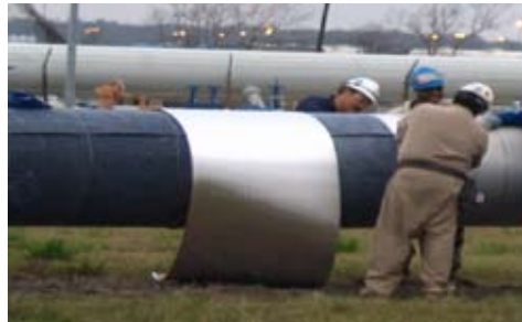
Steam Pipe Retrofits: Simple, fast installation of single-ply aerogel blanket overwrap can drive moisture out of old, wet insulation and recover system performance.
