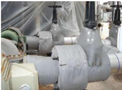
Removable Covers: Aerogel removable blankets are thinner, lighter, and last longer than conventional materials.
