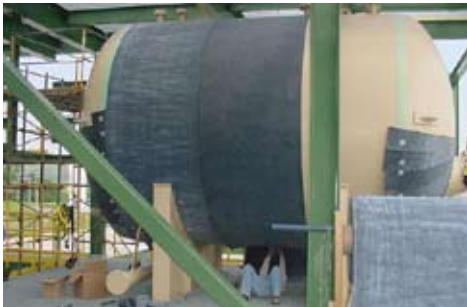
16' x 20' Vessel: Aerogel blankets increase labor productivity on tanks, towers, and vessels.
