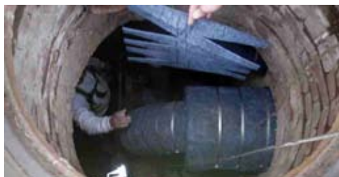
Tight Access Areas: Flexible aerogel blankets are ideal for tight access areas and can withstand periodic flooding.
